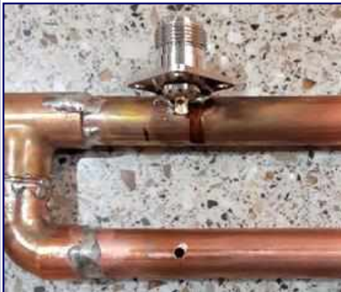
Figure 13 : Hole for Wire Drilled
