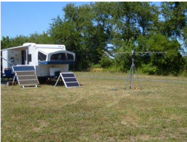
Above left: Satellite Communications Station
